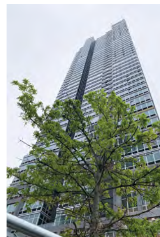
5203 CENTER BOULEVARD, HUNTERS POINT SOUTH, QUEENS (2021)
