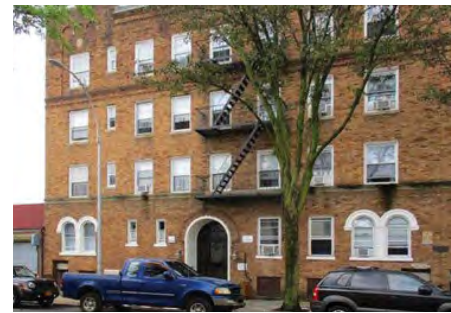
71-15, 71-21, 71-27 65TH STREET, GLENDALE, QUEENS (2019)
